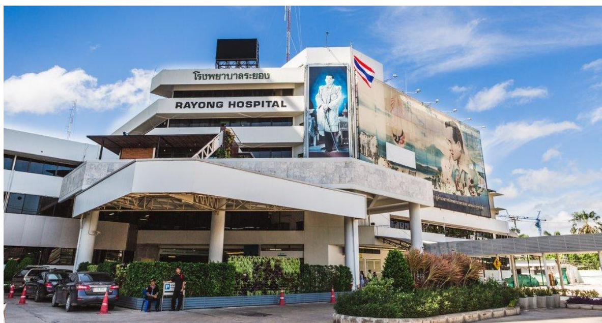
Figure 3-1. Rayong Hospital (Main Building). Source: https://www.rayonghospital.go.th
